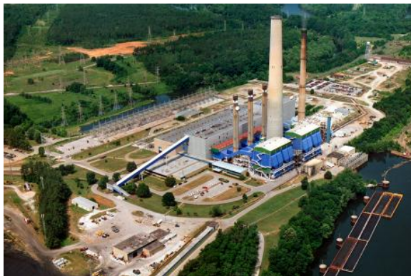
TVA Colbert Power Plant Huntsville, AL - DEC 1998
